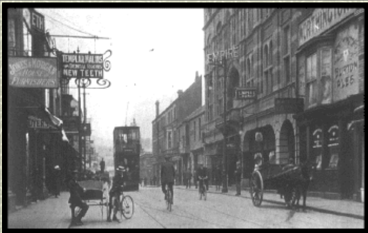
Oxford Street, Swansea, C1911
